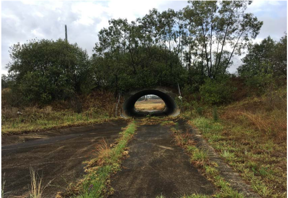
Photograph 5 - tunnel through embankment. Bow Bowing Creek is located below the concrete surface
